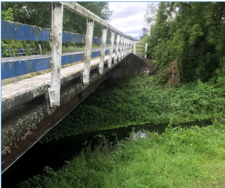
Figure 2.2: Kahahakuri Stream Bridge on Ongaonga Road
