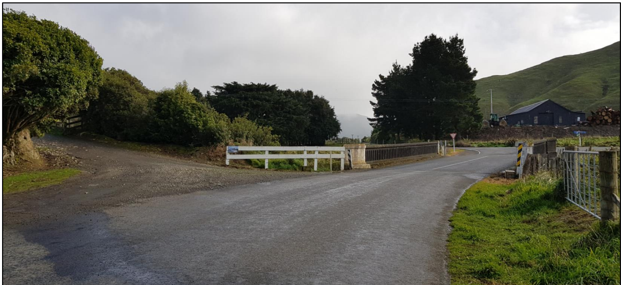
Figure 16 Internal Transmission line access (Opaki-Kaiparoro Road) and Makakahi River bridge
