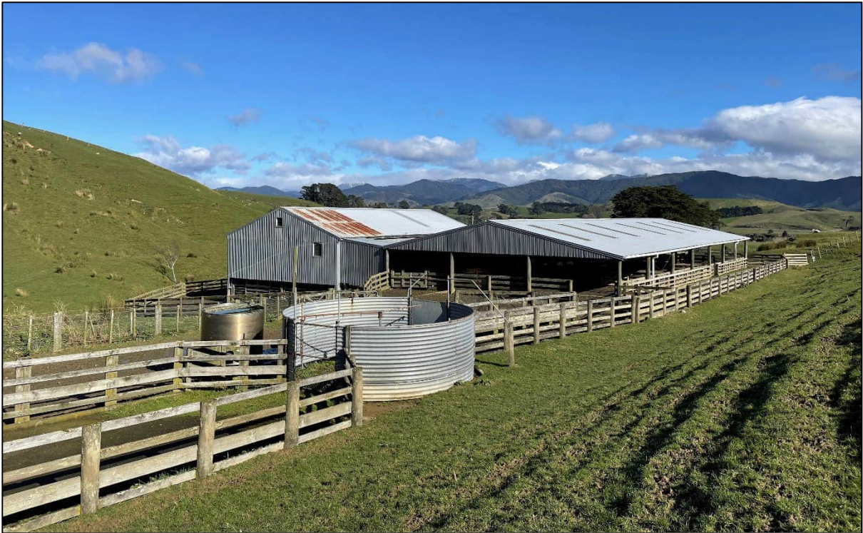
Photograph Appendix B.3: Woolsheds, stock yards and disused spray sheep dip and tank, looking south-west towards Old Coach Road.
