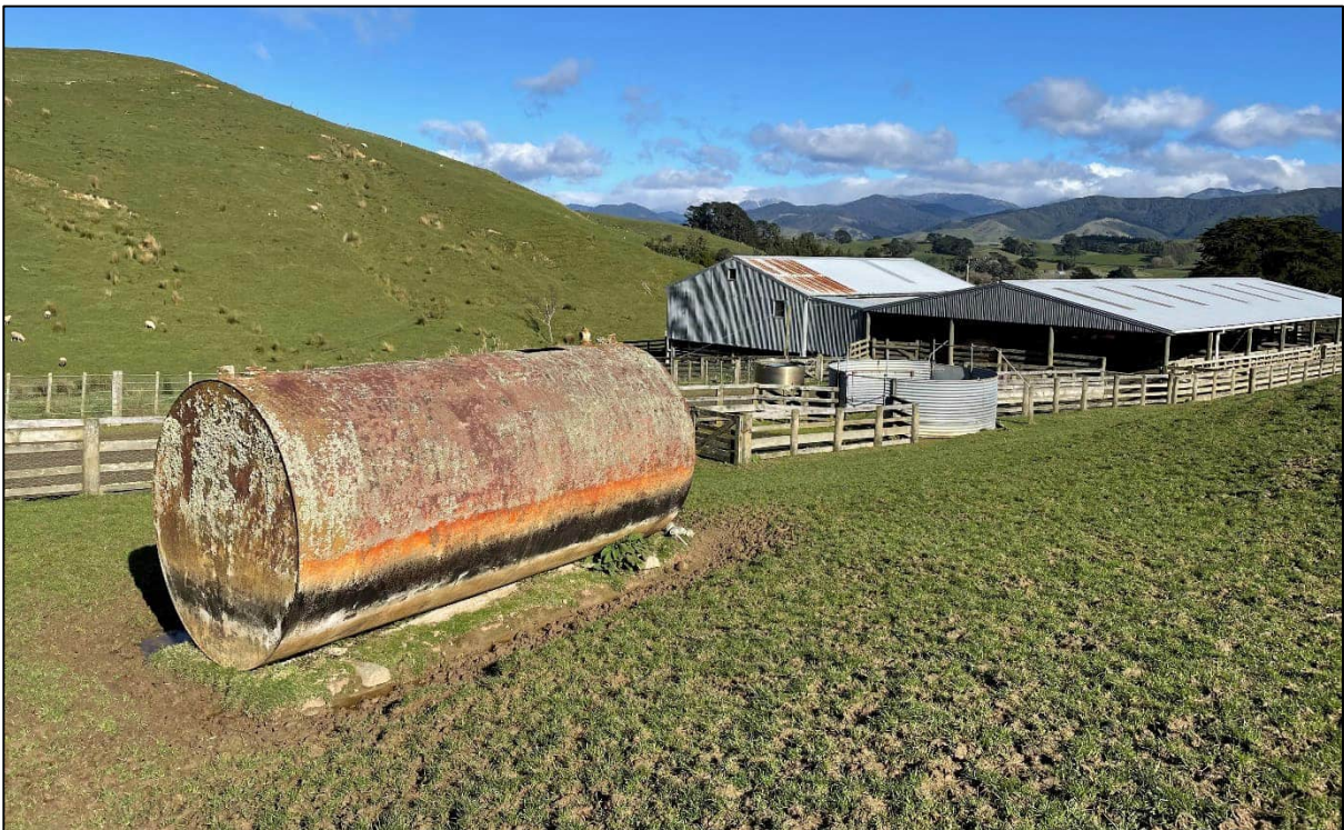
Photograph Appendix B.4: Aboveground storage tank, previously used for water storage present by northern woolshed.
